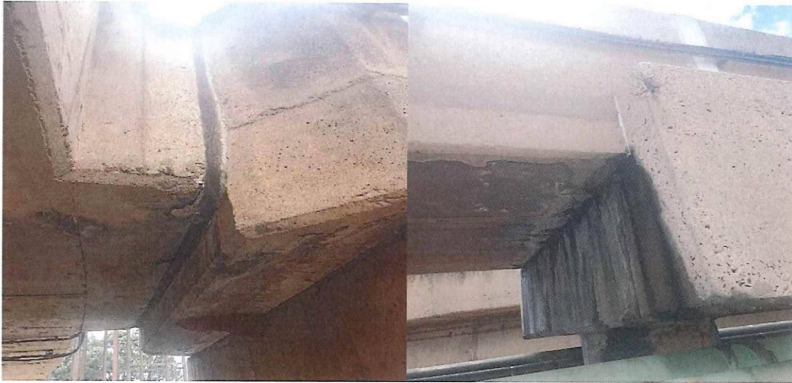
Figure 2: Leaks on Clarifier 48 launder construction joints
